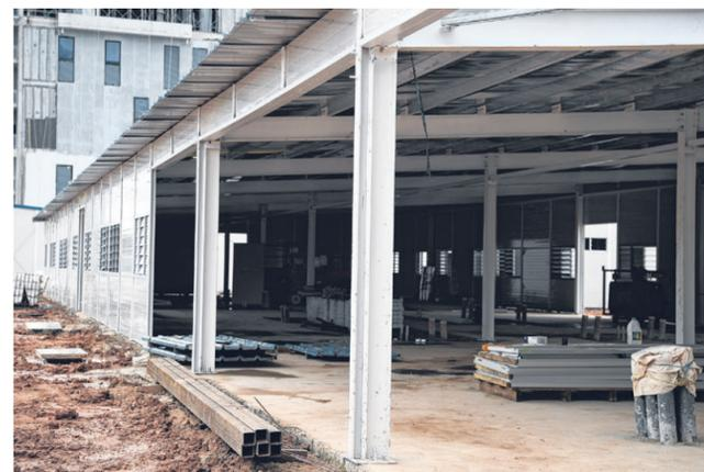
**1** After land at the site is excavated and prepared, a concrete foundation is laid. Steel columns and beams are put up, forming the structure of the dormitory block. To speed up the process of construction, prefabricated steel beams that are manufactured offsite and which can be quickly assembled at the site are used.
