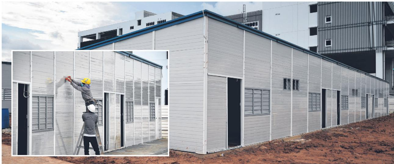
**2** External panels, which are also prefabricated, are added to the structure, forming the walls. A metal roof with insulating material is also added to keep the structure cool. Keeping the block to a single storey, instead of having multiple levels, keeps the structure light. This also helps to shorten the construction process as piling works do not have to be done to support a heavier structure.
