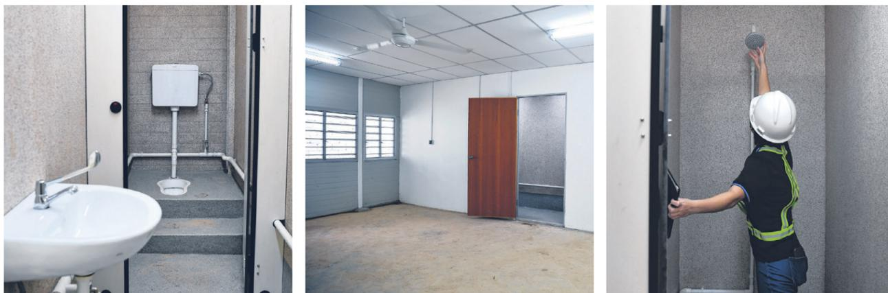
**3** The interior is fitted out with internal dividing walls and other amenities such as beds and toilets. The dormitory blocks have a modular design, meaning that the same design and construction process can be replicated for each block in the compound. In total, there are 20 blocks at the 2.5ha site. The QBD in Kranji Way will have shared facilities such as a canteen, a minimart, indoor recreational areas and multi-purpose hardcourts.
